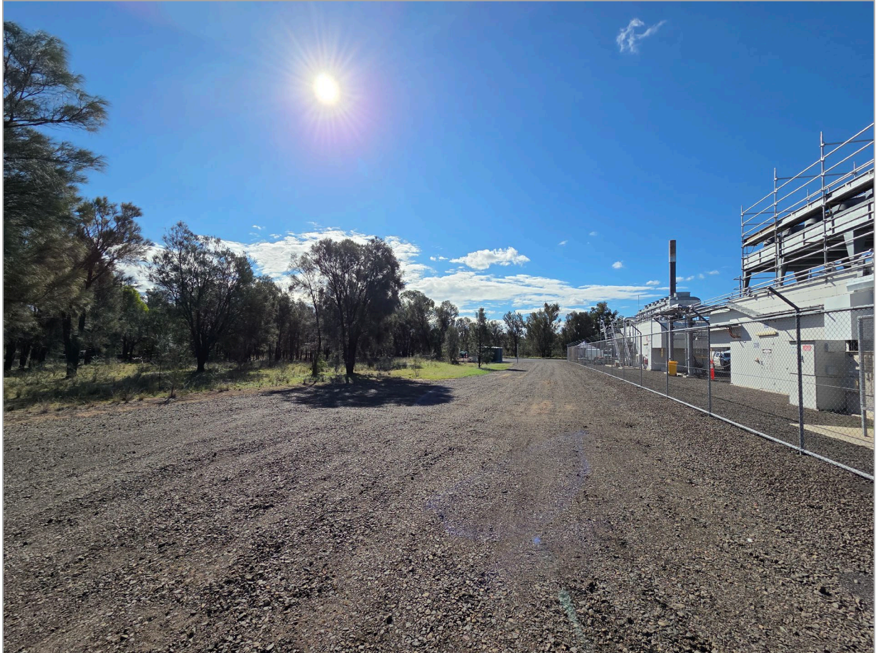
Photograph 1: Project site with Wilga Park Power Station to the east
